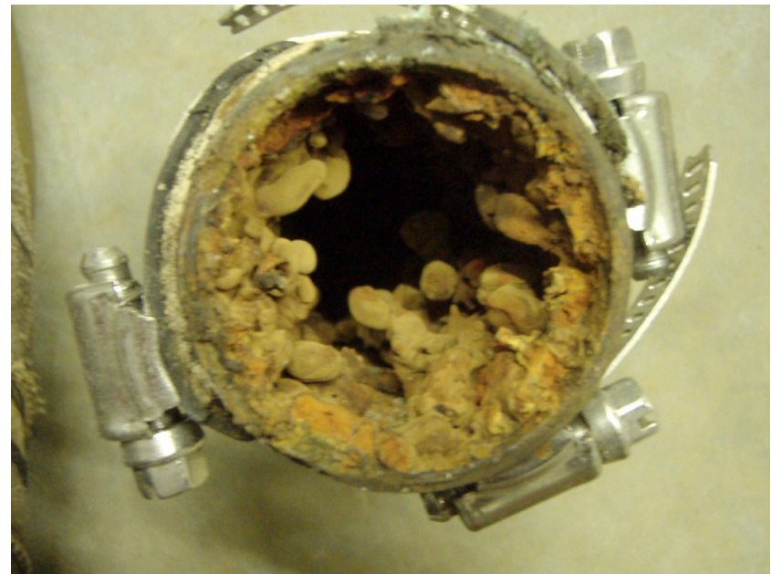
Old tank connection
